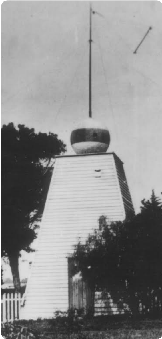
(left) The last of the Royal Observatory's time balls, dismantled around 1935. This one was located just behind the stables of the Main Building. (right) A repeating time ball controlled by an electrical signal from the Observatory was set up in the harbour in 1894 and is still there. Although the mechanism has been reconstructed, the Waterfront authorities are not prepared to hand-raise the ball each day for dropping.
