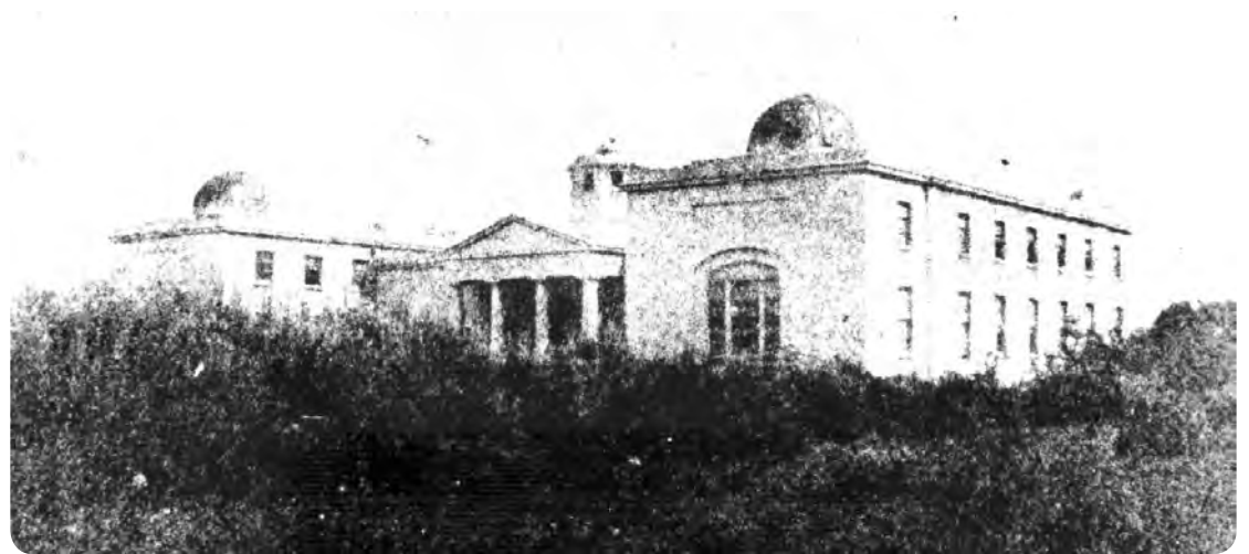
The Royal Observatory, Cape of Good Hope, in 1842 or 1843, seen from behind a hedge. This is the oldest photograph of any observatory and is one of the first photographs taken in South Africa. The photographer was Charles Piazzi Smyth (see page 14).
