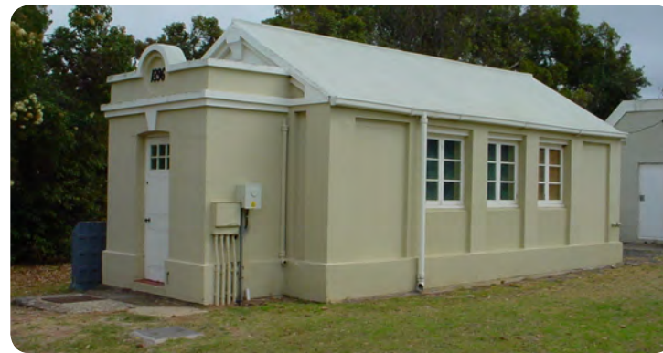
The Battery House (1896 Building) next to the McClean, contained lead-acid batteries that were charged during the day by a steam-powered generator.
